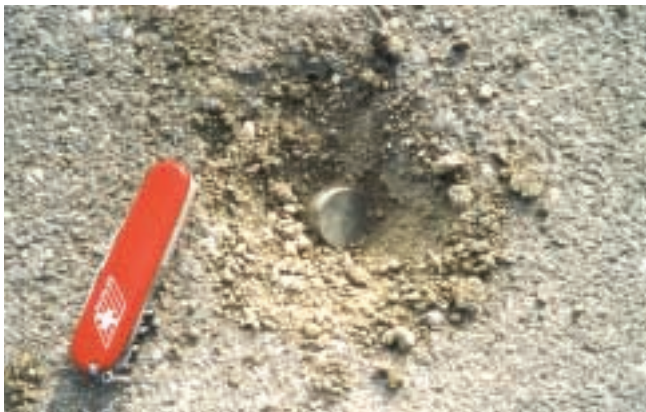
The jacket remained in the hole and the penetrator continued into the soil beneath the asphalt layer.
