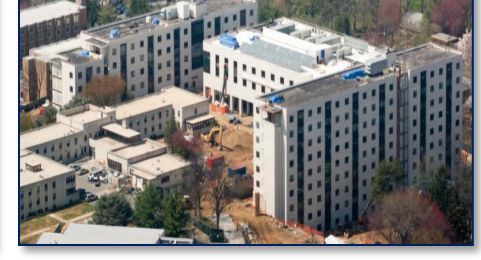
Building 62: Barracks/Dining/Admin 8 floors; 295K sqft; ECD: June 2011
