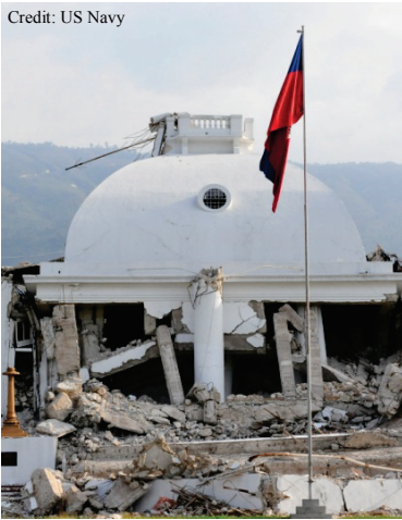
Figure 6-1: The Collapsed Presidential Palace of Haiti
